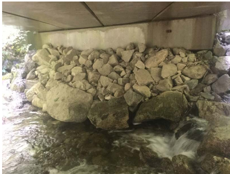
Right Bank Abutment when facing downstream
