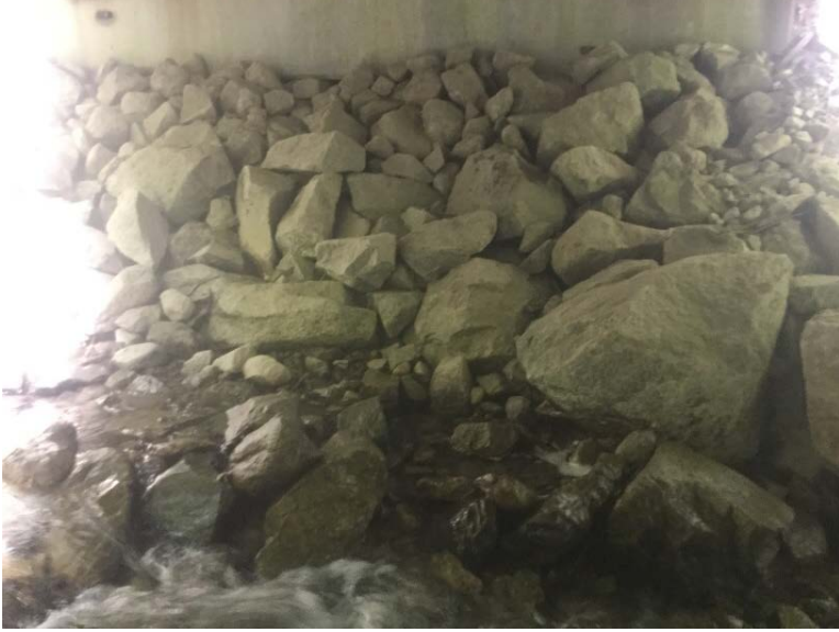
Left Bank Abutment when facing downstream
